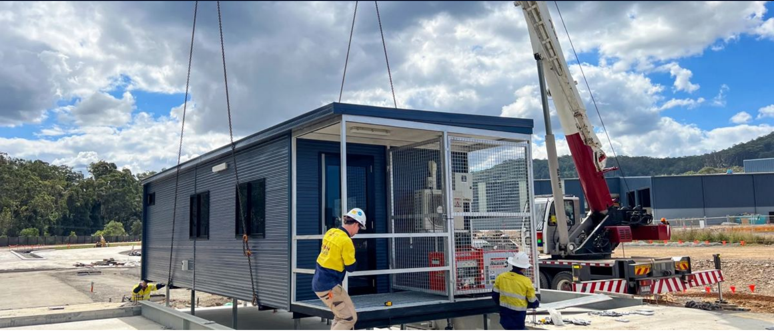
Building placement during installation. Multitrade Group project photography.
